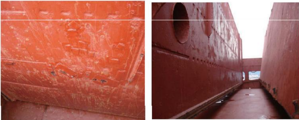
4-1 Holed hatch covers, attention to be paid to the lower part of the cover panels and the ventilators or cement holes in panel (if any)
